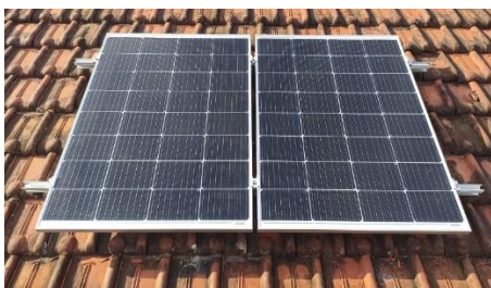
Gambar 3. Hasil Instalasi Panel Surya
